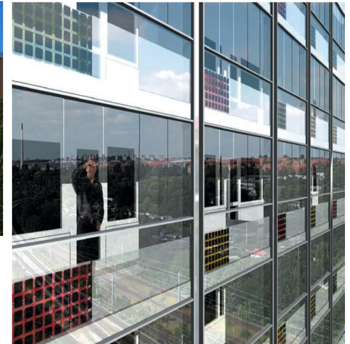
Glass facade with integrated photovoltaics towards the busy street
