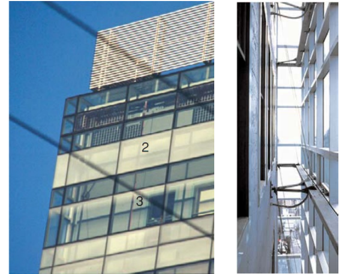
PV double skin façade (source: tboake.com)
